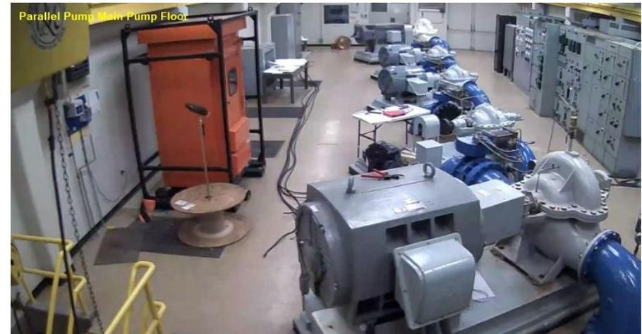
**Four pumps provide total potential capacity up to 40 MGD**
