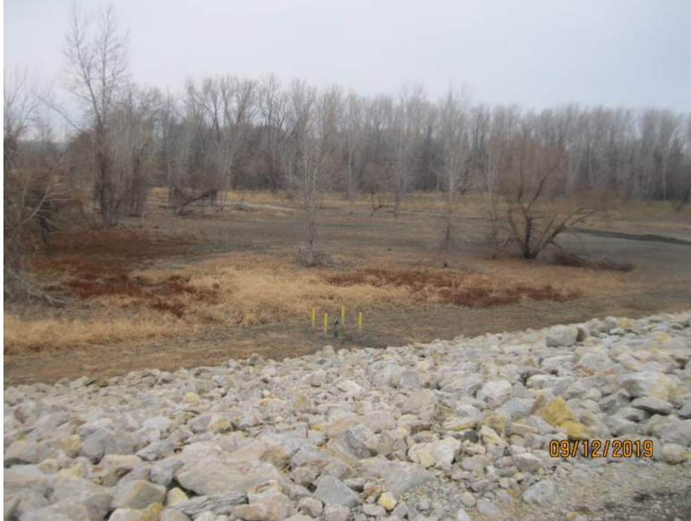
Figure 4 – Rip Rap on Exterior North Dike of Bottom Ash Impoundment
