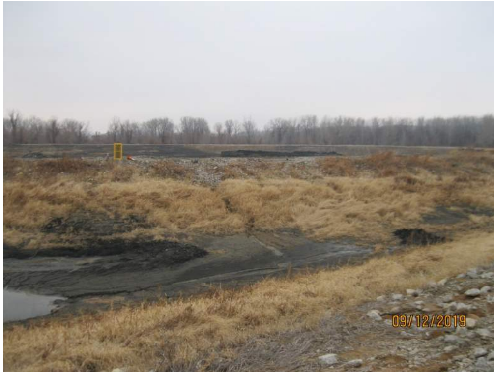
Figure 3 - Interior Slope of Clear Water Pond without Rip Rap.
