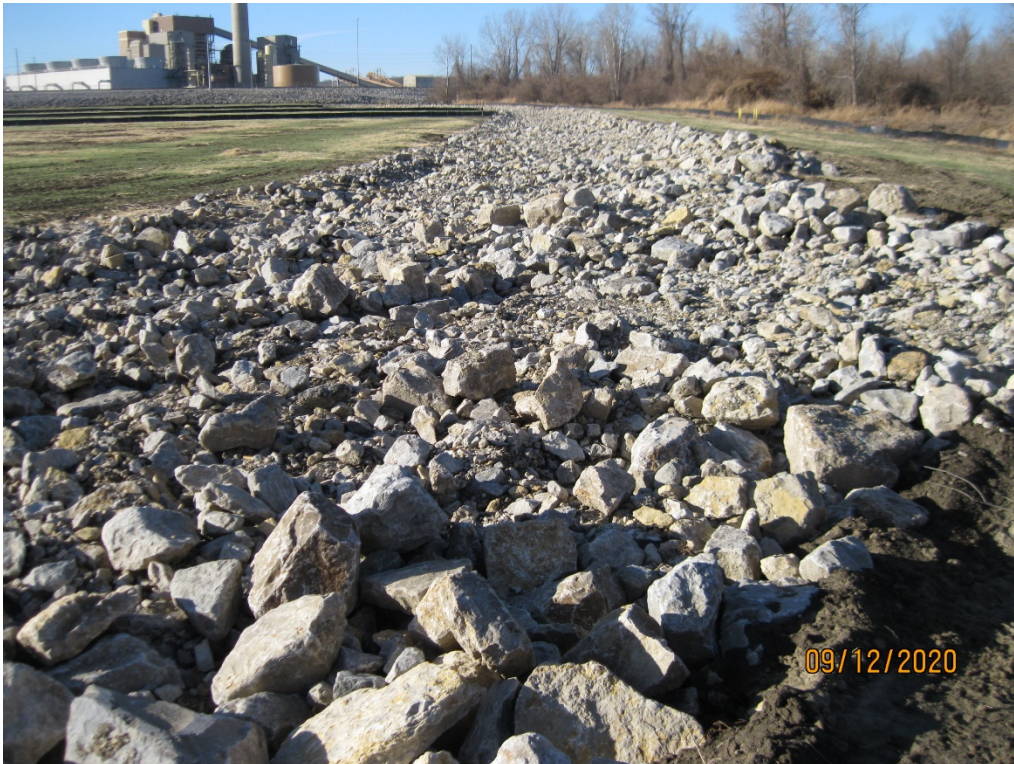
Figure 2 – Previous Location of Discharge Structure
