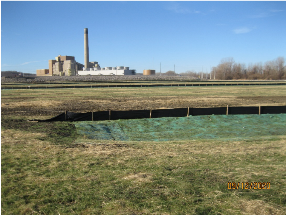
Figure 3 – Graded impoundment area – From east looking northwest.
