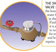
THE SHUT-OFF VALVE inside the house controls water flow in the home. Find out where it is and how to turn it off for emergencies and home repairs.
